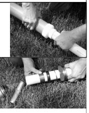
DO NOT put gasket over lock ring. This may cause a leak or pullout.
